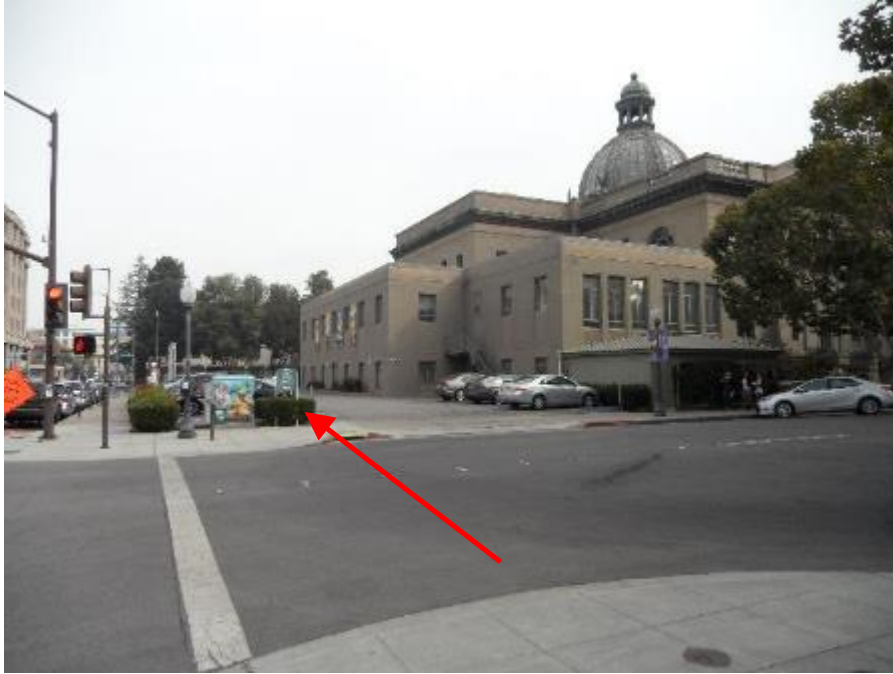
Rear quarter view from Hamilton and Marshall Streets. Lathrop House is proposed to be relocated on parking lot.
