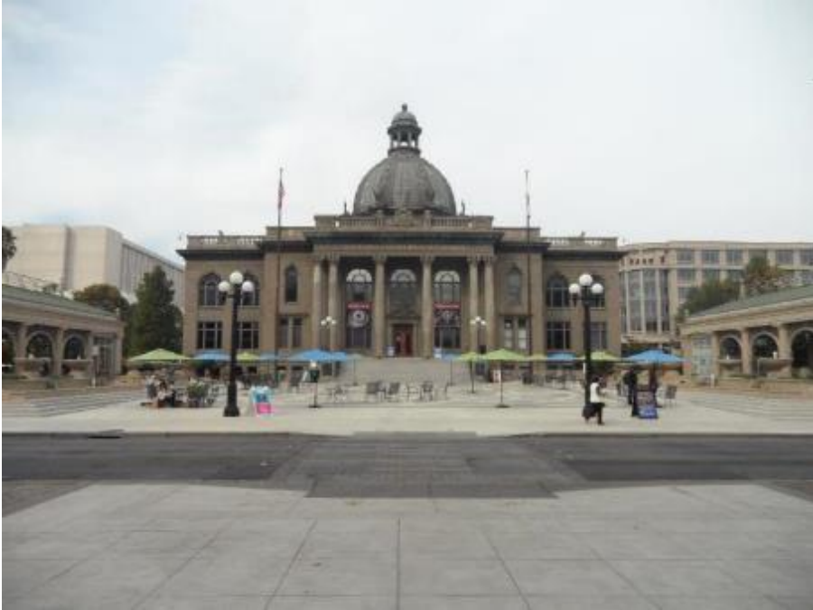
Broadway façade flanked by pavilions.
