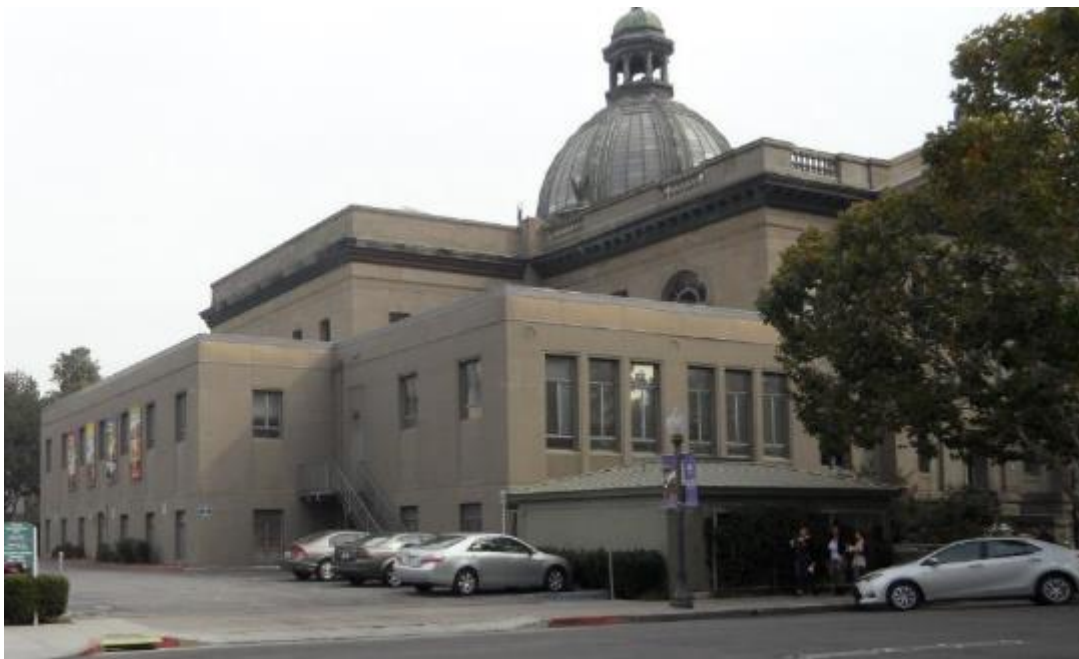
Closeup of rear addition.
